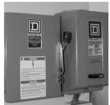
Figure 9-1 Power switch for machines with coolant-through-the-spindle option.
